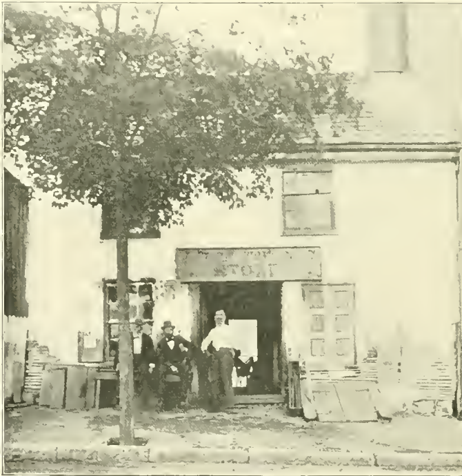
CALEB TAYLOR'S STORE—THE OLD EST HOUSE IN THE TOWN.
